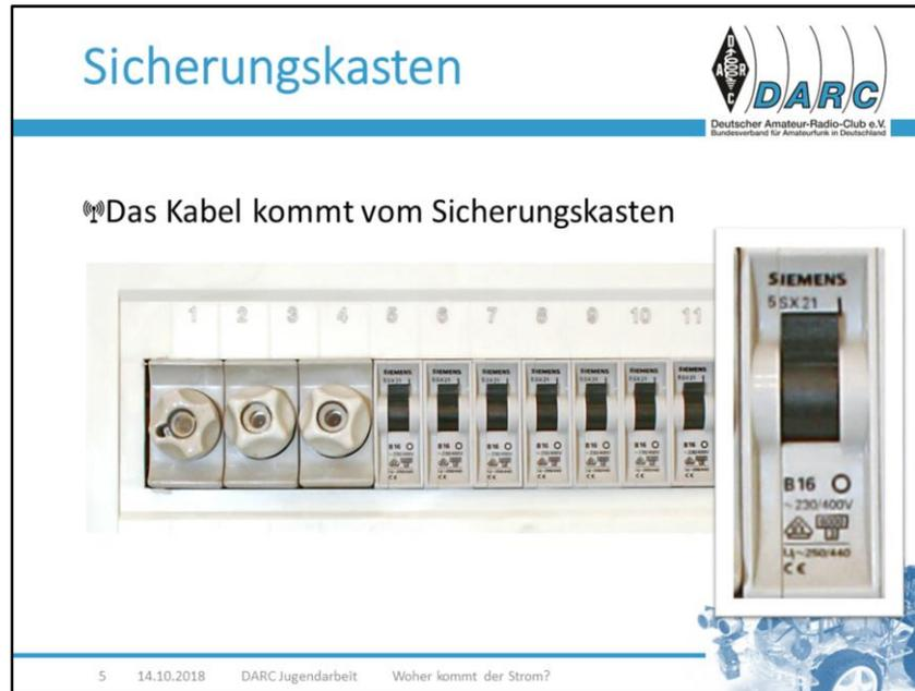
The slide is titled 'Sicherungskasten' (Circuit Breaker) in blue text. It features a photograph of a row of circuit breakers in a rack, numbered 1 through 11. A callout box on the right shows a close-up of a Siemens B16 circuit breaker, which is a 16A, 230/400V breaker. The slide also includes the DARC logo and text in the top right corner. At the bottom, there is a footer with the text '5 14.10.2018 DARC Jugendarbeit Woher kommt der Strom?'.
